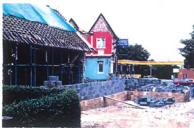
...the rear of Millington Hall
