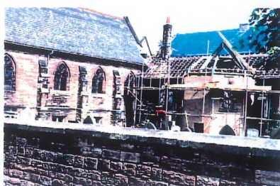
...the apse under construction
